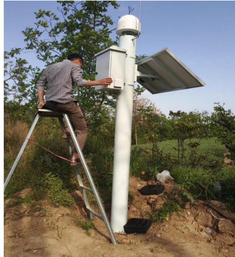
Monitoring station debugging
